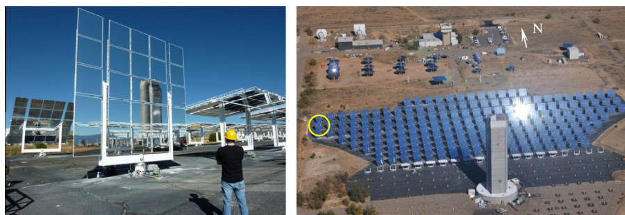
Fig. 1. Left: heliostat 12W14 at the NSTTF in Albuquerque, NM, which was retrofitted with 3M™ Solar Mirror Film 1100. Right: NSTTF heliostat field with location of 12W14 heliostat circled.
